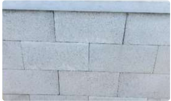
Above: a sample wall of dry stacked, mortarless blocks; steel reinforced and grouted solid, using our precision interlocking concrete blocks.
